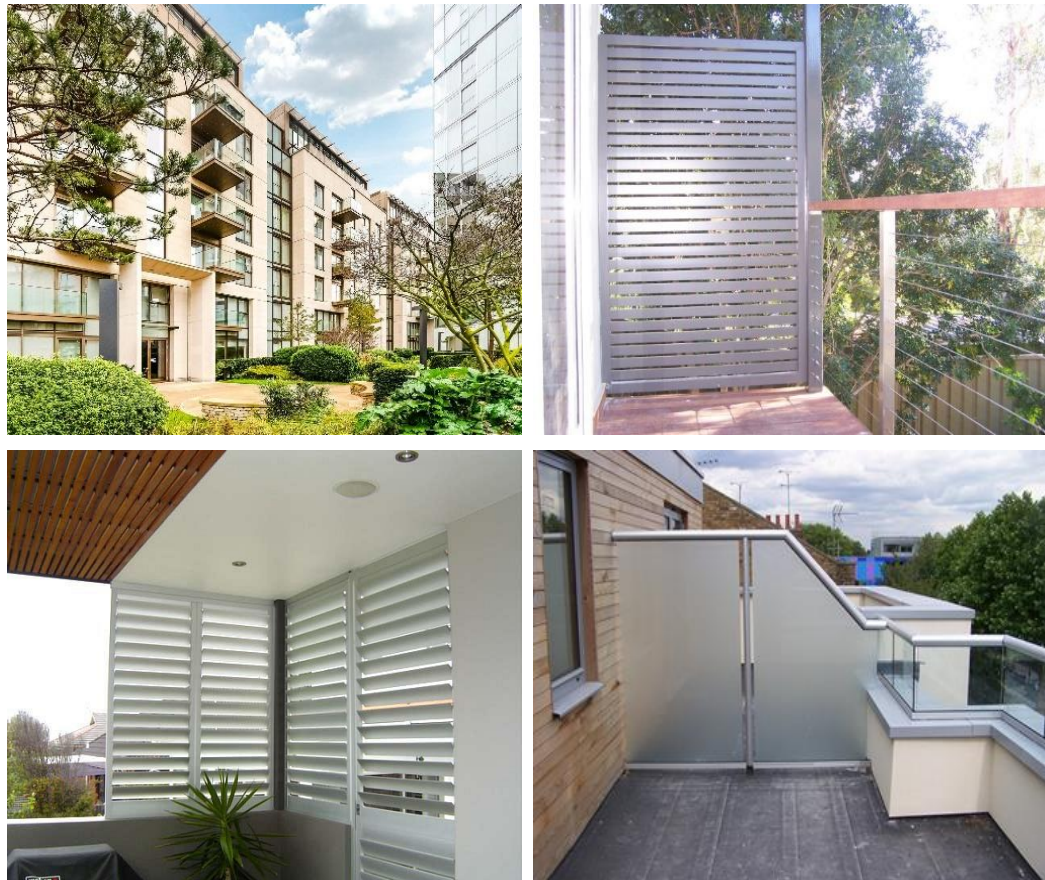
Figure 20: Example mitigation measures for private balconies
