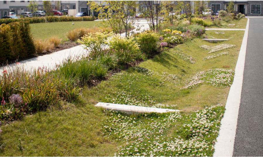
Grass swale with Check Dams for sustainable drainage; Greystones, Co. Wicklow, by Cairn.
