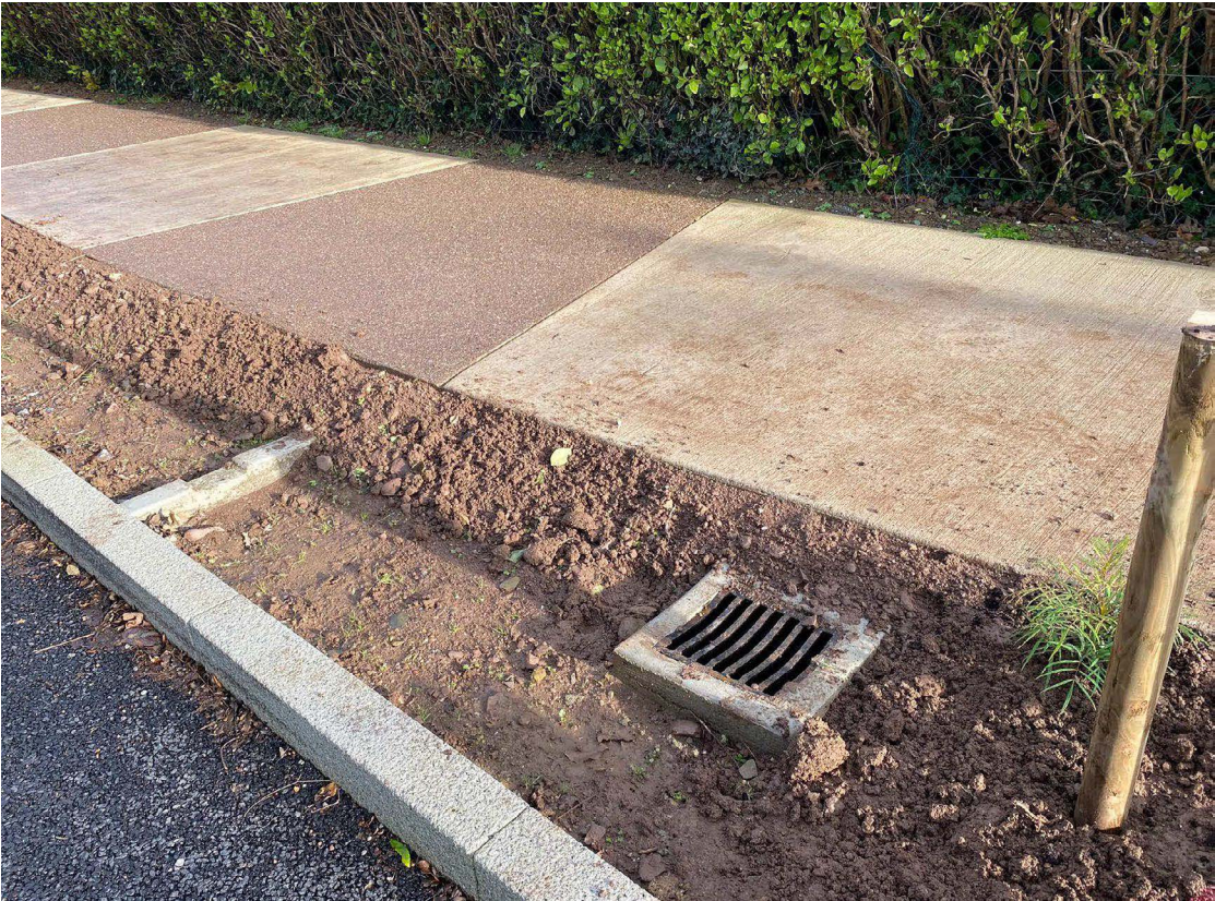
Example of check dam and overflow gully within a linear rain garden on a fall; Belgooly National School, Cork.
